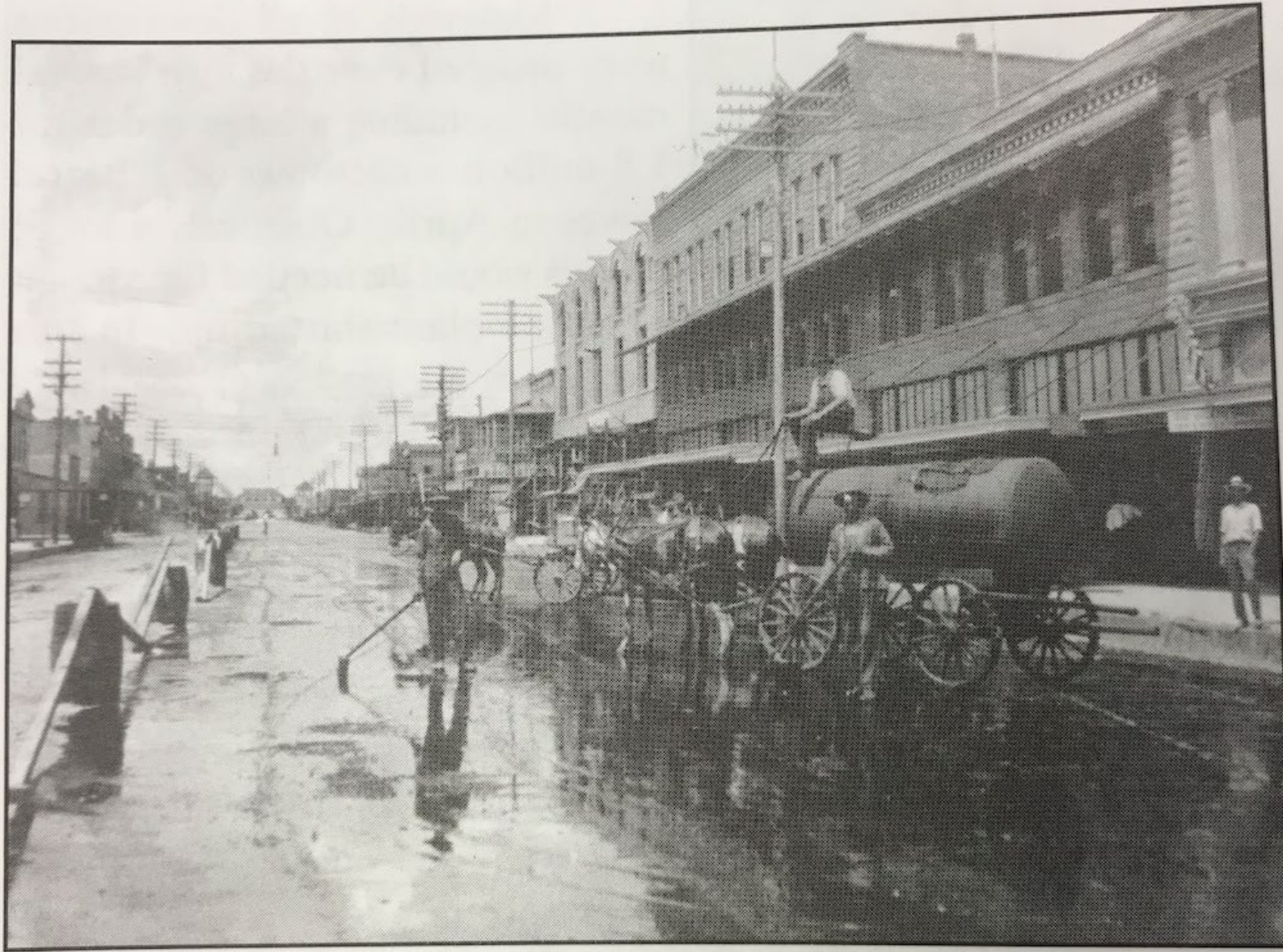
Paving Proctor Street in Port Arthur in circa 1908 with Texaco asphalt from PNW.
