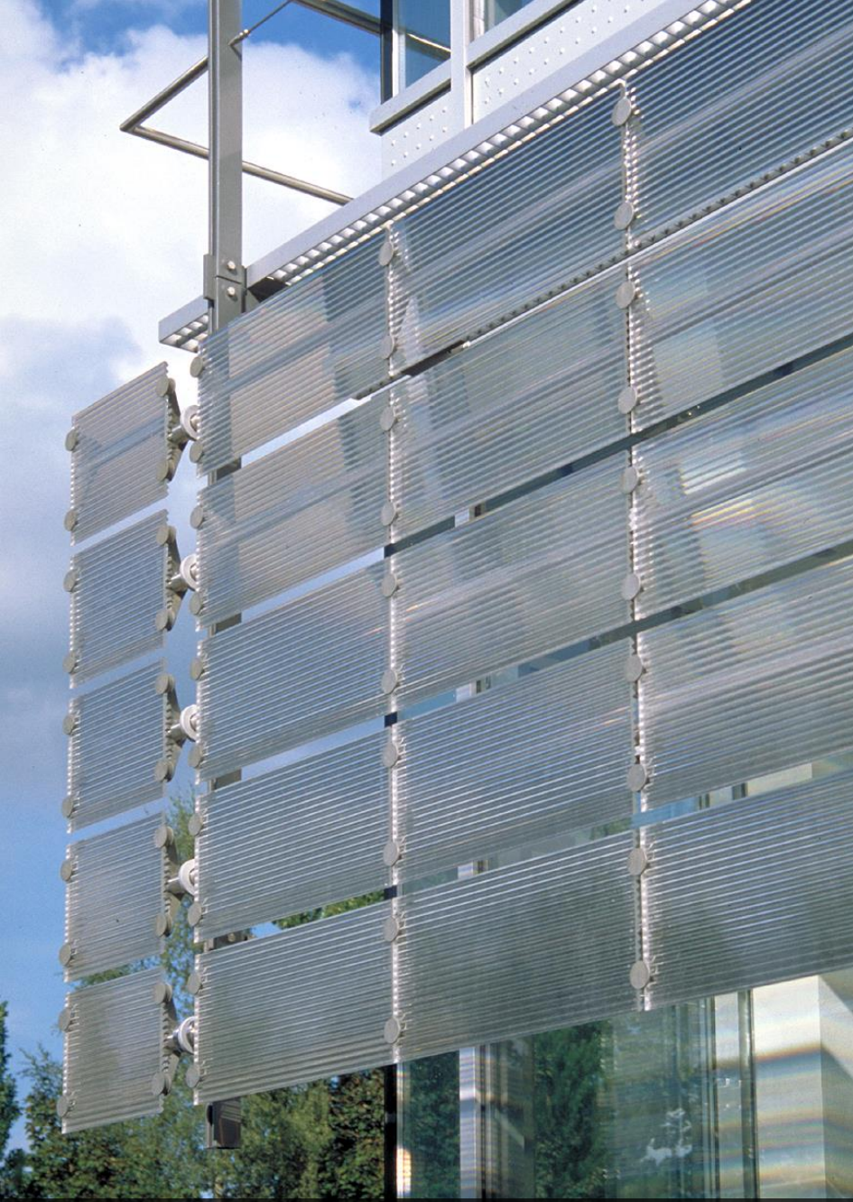
Direct/passive use of solar energy: Adaptable facade/Use of daylight Redirection of daylight with deflecting prisms
