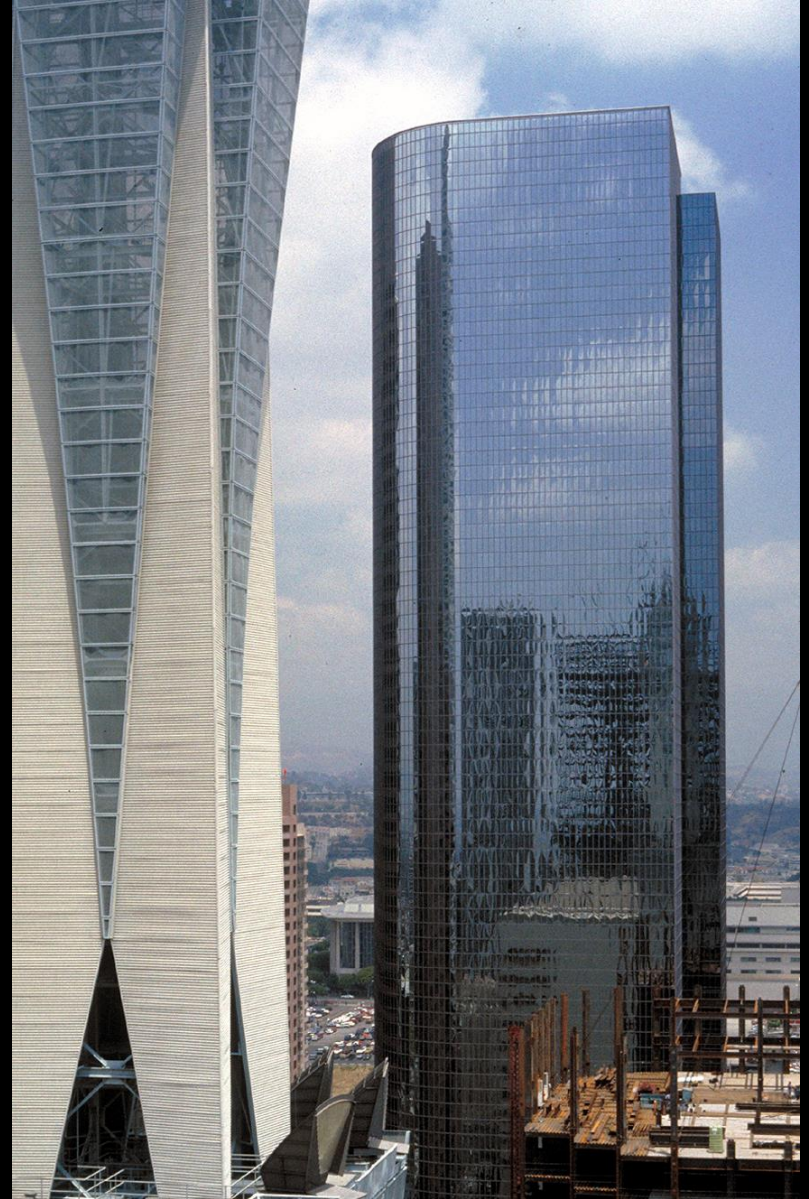
Administration Building Los Angeles, Two California Plaza, 1992, Arthur Erickson
