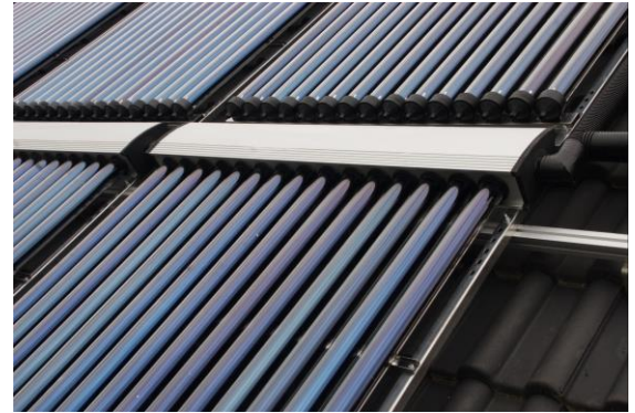
Heat pipe/vacuum tube collector
